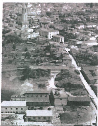
Vista general de la fàbrica Reliablé (Reliable S.A.)
